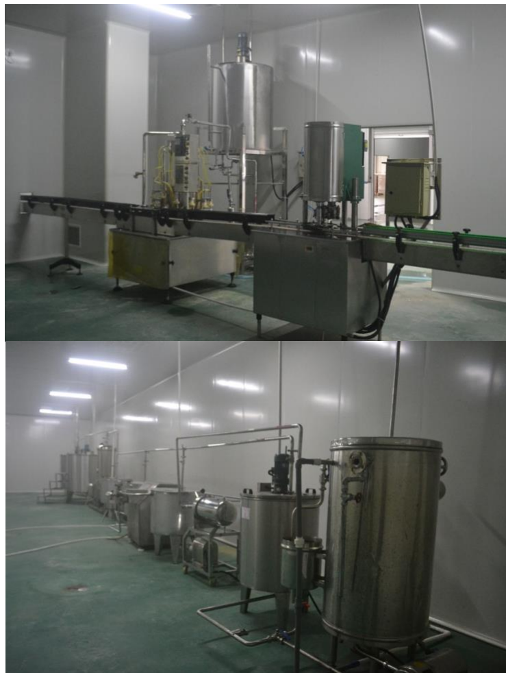
Figure 1: Installation and commissioning of new vinegar beverage production line
